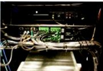
Shown here is an example of multiple copper-based signals combined onto a unified fiber-optic routing and transmission platform.
